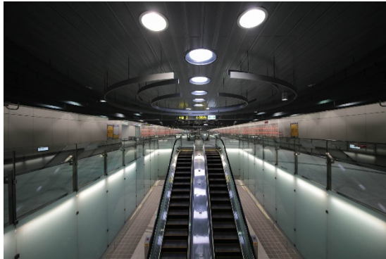
Figure 28: Solar Tubes at Dingpu Metro Station (Source: J.J. Pan & Partners)
