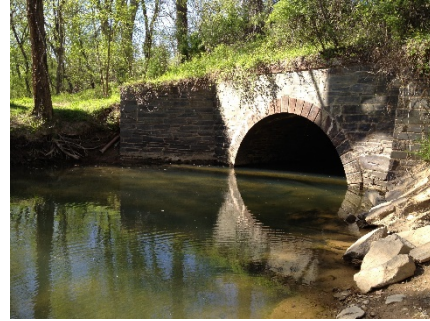
Figure 51: Culvert north of Pennyfield Lock (Source: Author)
