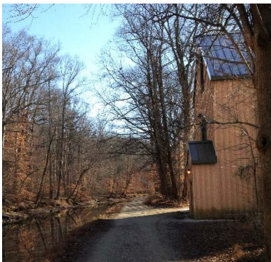
Figure 54: Pump Station for Rockville water supply, near Swains' Lock (Source: Author)
