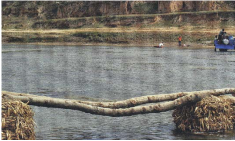
Figure 41: Original Bridge (Source: Edward NG)
