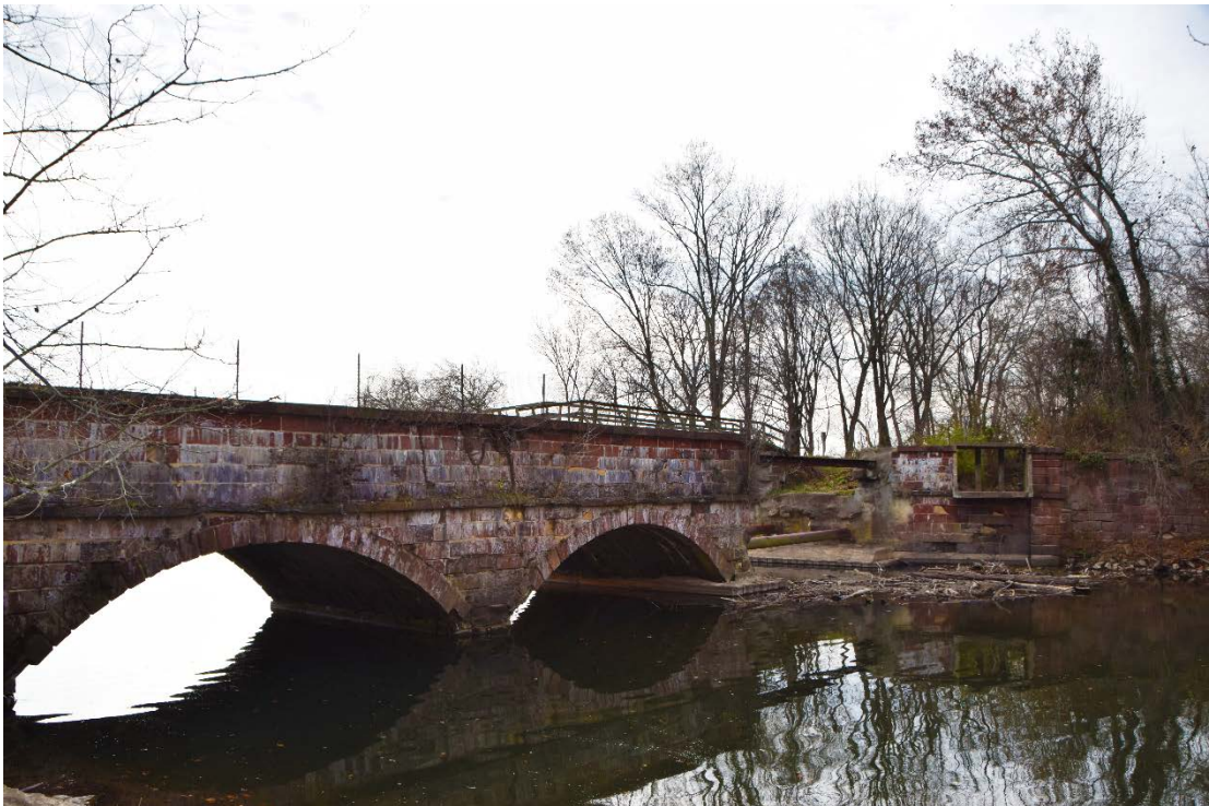
Figure 59: Seneca Aqueduct (Source: Author)
