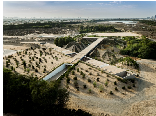
Figure 13: Wasit Natural Reserve (Source: X Architects)
