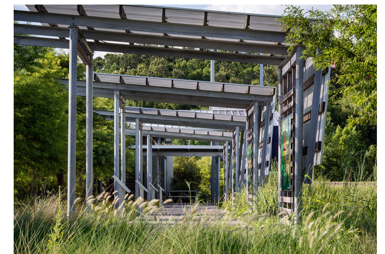
Figure 4 : Main Entrance and Rain gardens (www.asla.org)
