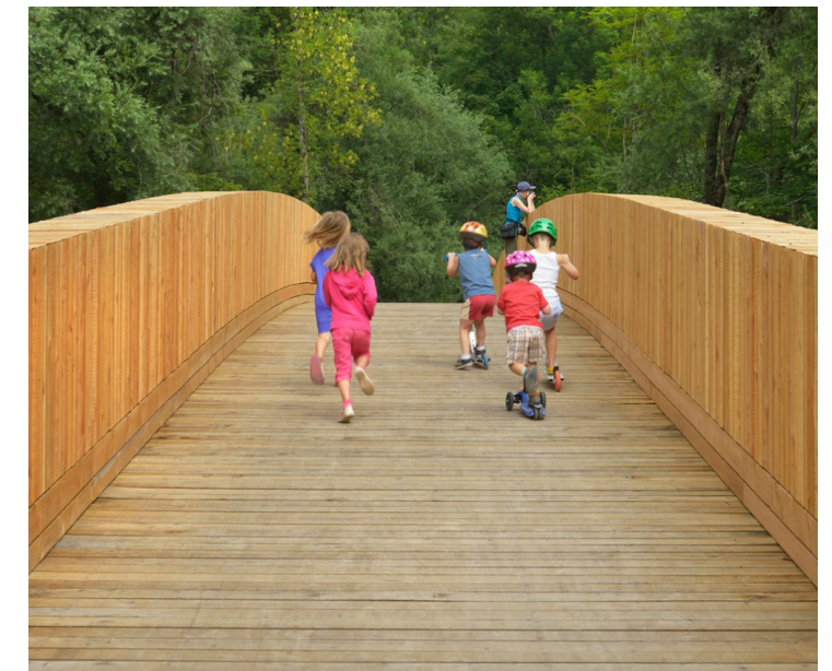
Figure 4. Arched Foot Bridge (www.inhabitat.com) Example of bicycle and foot bridge, DANS Architects used timber planks and shingles to create this 54 long meter arched foot bridge, Slovenia (Nicole Jewell,2015)
