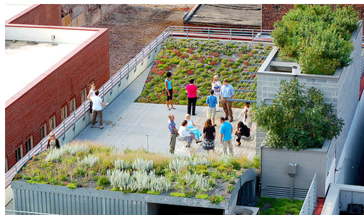
Figure 1. ASLA Headquarters Green Roof A green roof located on the new headquarters of the American Society of Landscape Architects in downtown Washington, DC. The roof is intensive in some areas and extensive in others. (www.asla.org)
