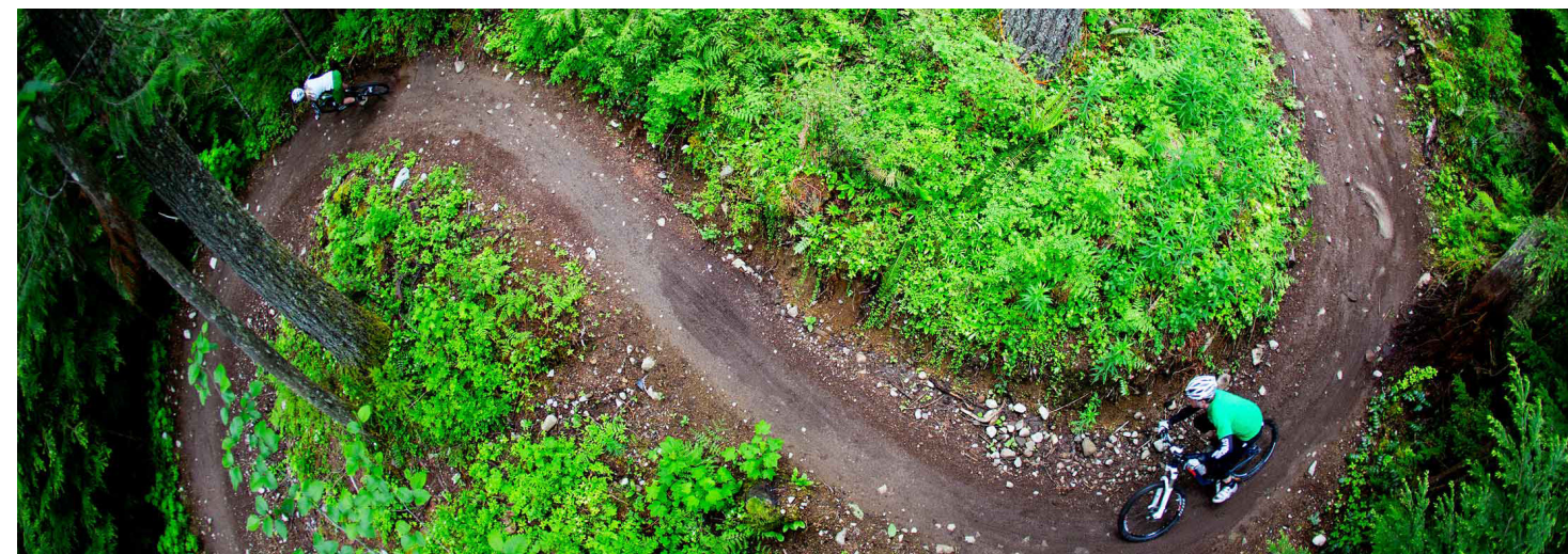
Figure 3. Switchback (www.exploresquamish.com) Switchbacks are ideal for mountain bikers and hikers. This trail element works well with vegetation and rocks along the tread to reduce the occurrence of users from cutting through ecologically sensitive areas.
