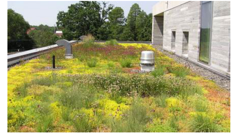
Figure 3. Extensive Green Roof An extensive green roof located at Swarthmore College, Swarthmore, Pennsylvania. Extensive green roofs support smaller vegetation that does not need much water or maintenance, such as sedums. (www.greenrooftechology.com)
