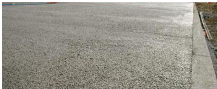
Figure 2. Pervious Concrete ( www.perviouspavement.org )
