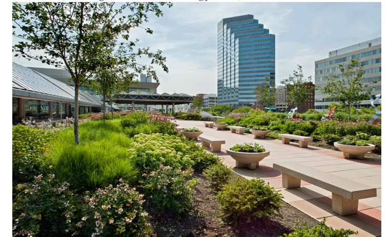
Figure 4. Intensive Green Roof An intensive green roof located at the Baltimore Convention Center. Intensive green roofs support larger vegetation, even trees. (www.greenroofs.com)
