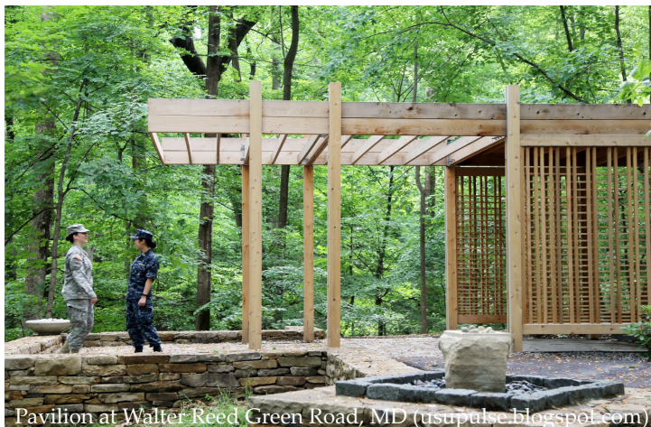
Pavilion at Walter Reed Green Road, MD (usupulse.blogspot.com) Figure 10. Pavilion at Walter Reed Green Road, MD (usupulse.blogspot.com)
