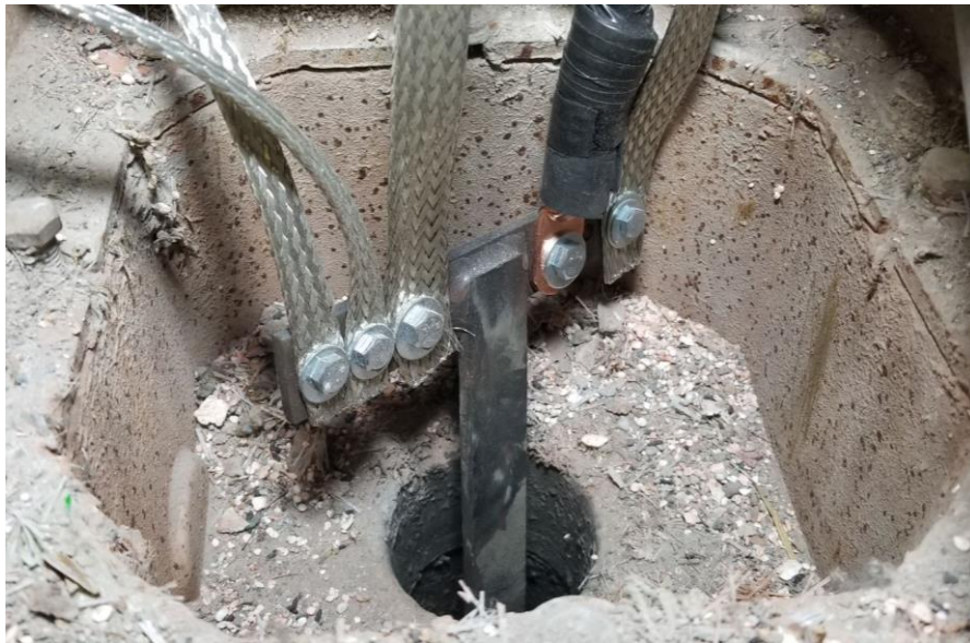
Figure 70: Earth ground. The test frame, positive welding lead, all of the EMI shielding, and the Galil controller body were attached to earth ground.
