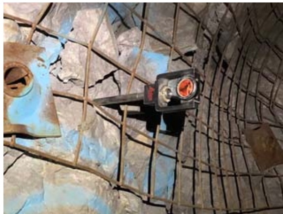
Figure 10. Reflector installed on the mine rib at a known coordinate (on the local mine grid) that is used for determining the total station location by performing a resection.
