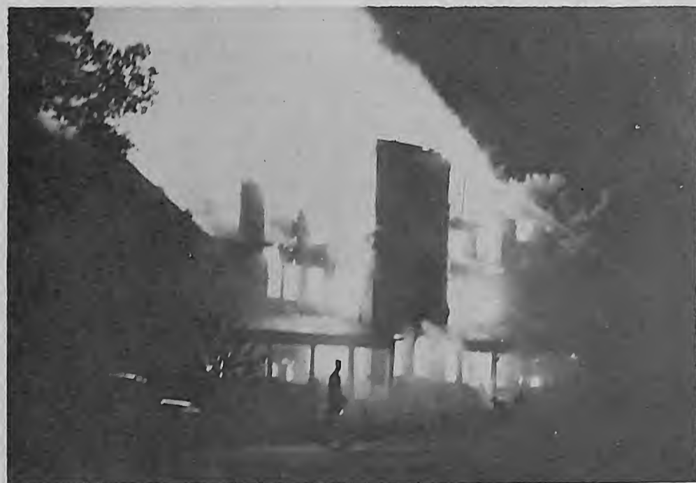
1957 - Huggins-Curtis Building burns - Possible electrical short.
