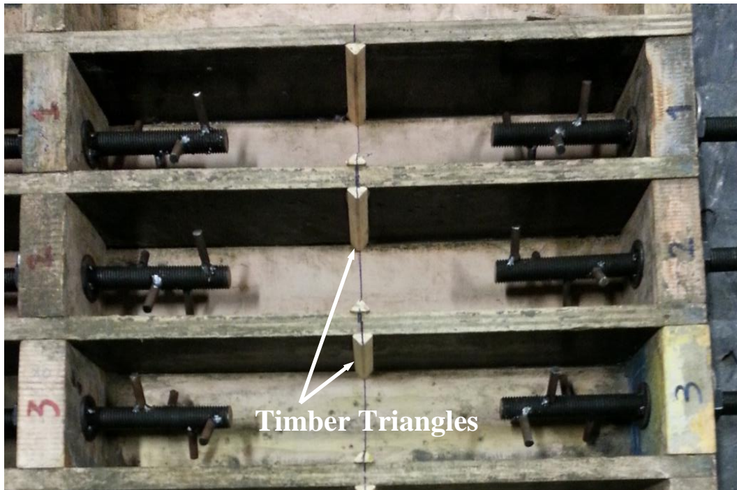
Figure 2.3: Completed formwork for the casting of the SCC specimens
