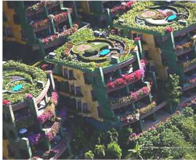
Figure 6 Vegetation canopy solution, by planting/cultivation native-green covers on top, sides and around buildings within high-temperature regions.
