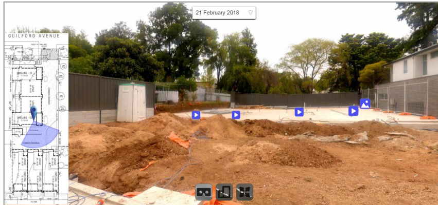
Figure 4: Concrete pouring virtual tour of Guilford Avenue property building site
