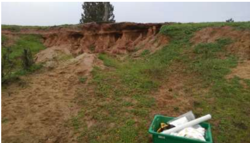
Figure 60: Overview of sample site Gala Vale 'south'.
