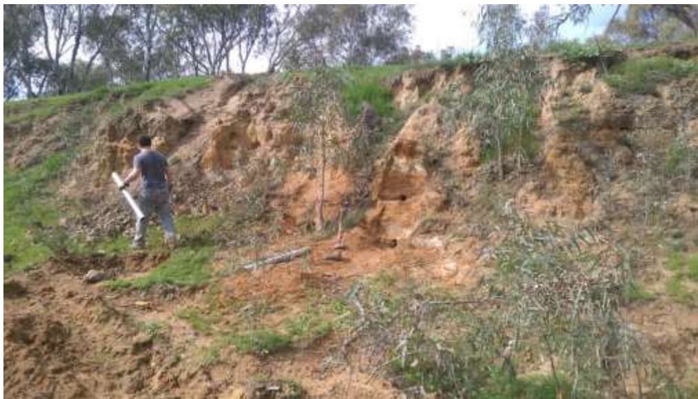
Figure 77: Overview of sample site Thurrowa Road.
