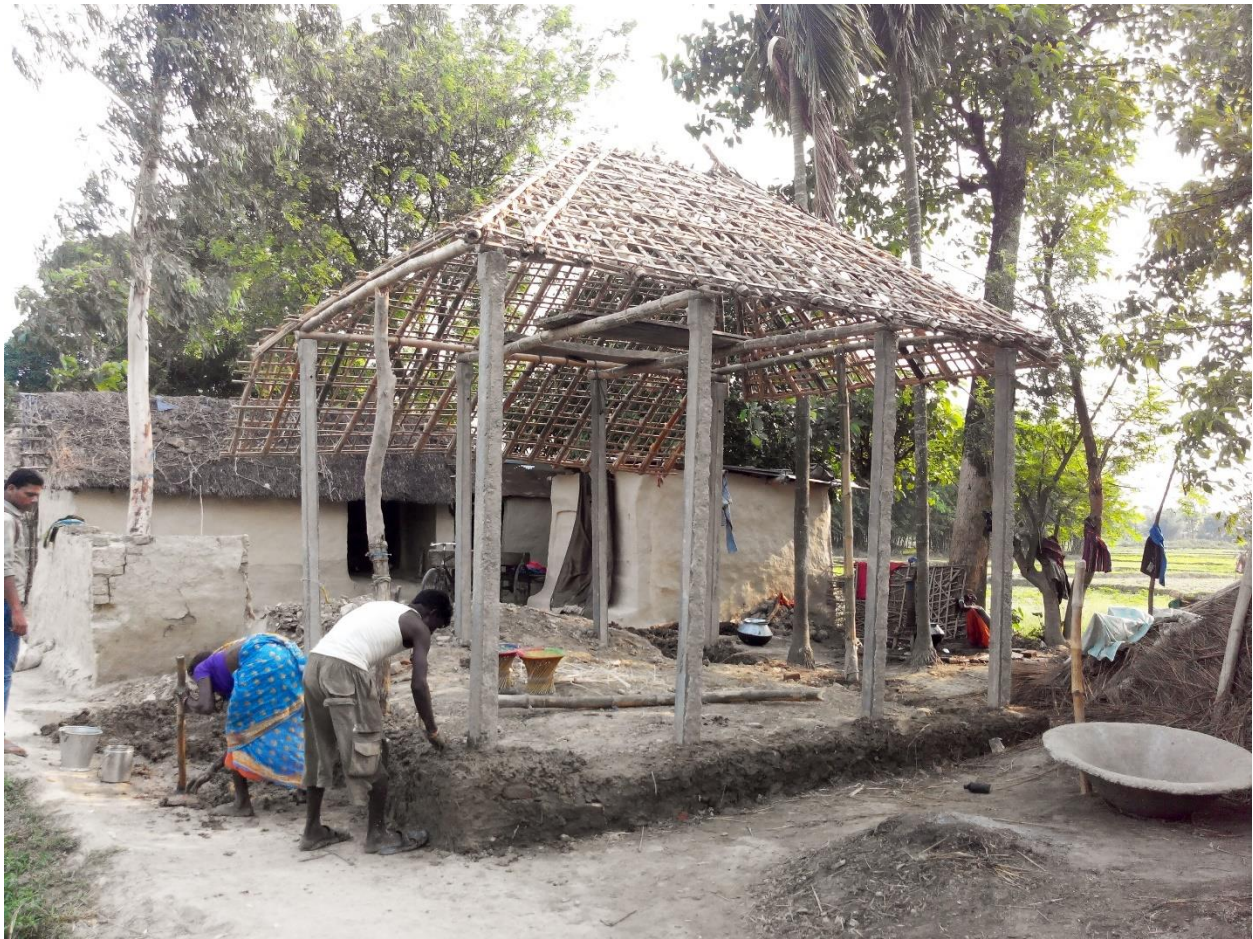
Photograph 6.9: A family engaged in constructing a house in Musahari Tol, Joginiya
