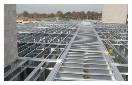
FIGURE 1.1. Cold-formed framing system (image courtesy of ClarkDietrich Building Systems)
