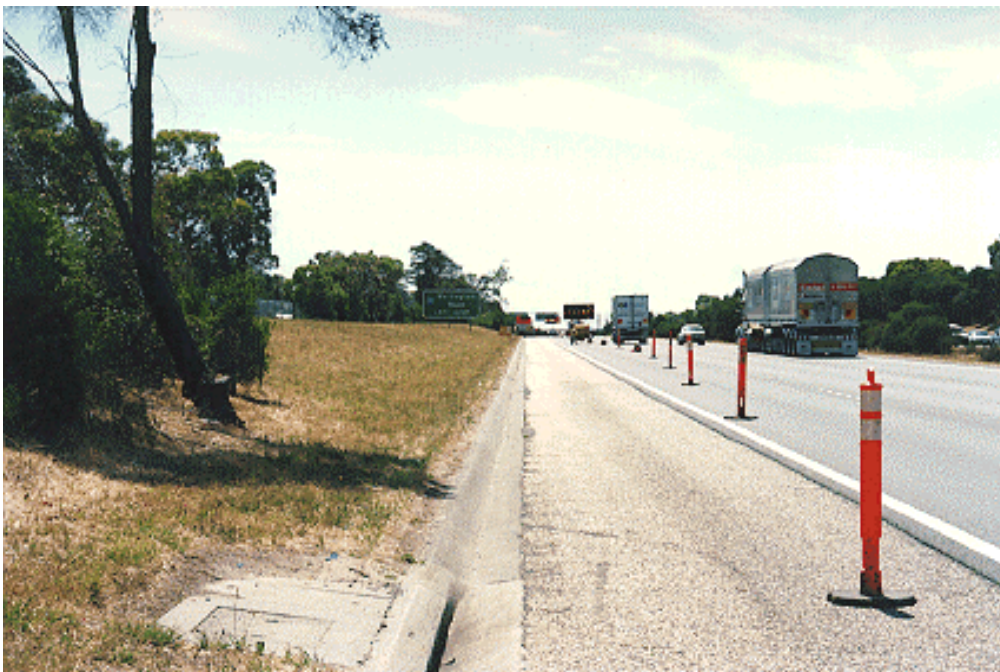
Figure 6: Traffic Management in the Work Zone
