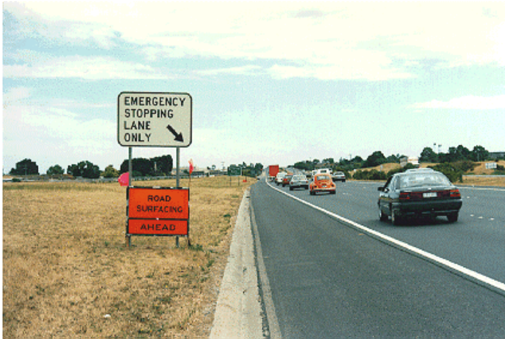
Figure 3: Advance Warning Static Signing
