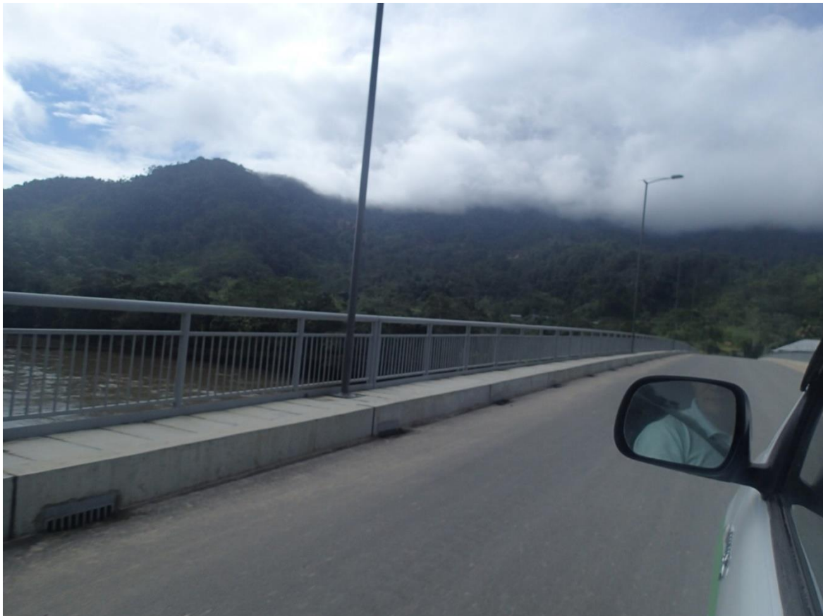
Figure 8: Newly constructed bridge on the road to Yanua and Churubia
