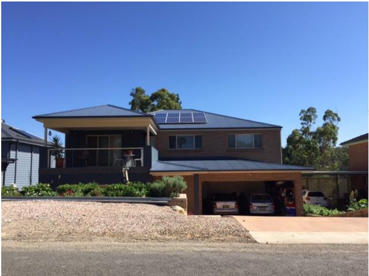
Figure 5.5 A rebuilt home with solar panels in Winmalee
