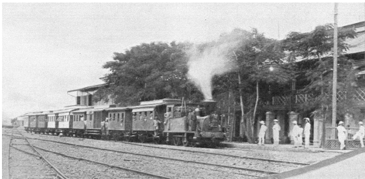
Figure 75: A train at a station in Bangkok during the reign of Rama V. 69
