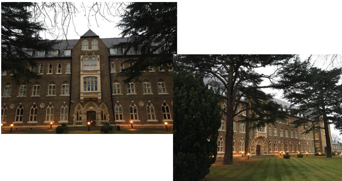
Figures 59 and 60: Lancaster House, Borough Road, Osterley, London was part of Borough Road College between 1889 and 1976. In 1976, Borough Road and Maria Grey teacher training colleges were merged into the West London Institute of Higher Education. During the late 1990s, the Institute became Brunel University. In 2006, the University sold Lancaster House, and it is now used as private flats. 54 These pictures were taken by the researcher in December 2016.
