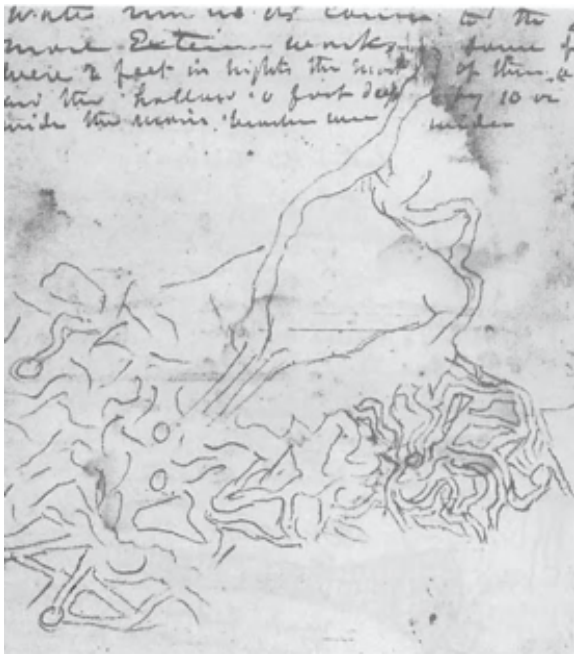
Fig. 68 George Augustus Robinson's sketch of an Aboriginal drainage system at Mount William. This sketch depicts just over half of the six-hectare maze of artificial channels he described by Robinson (Source: Mitchell Library).
