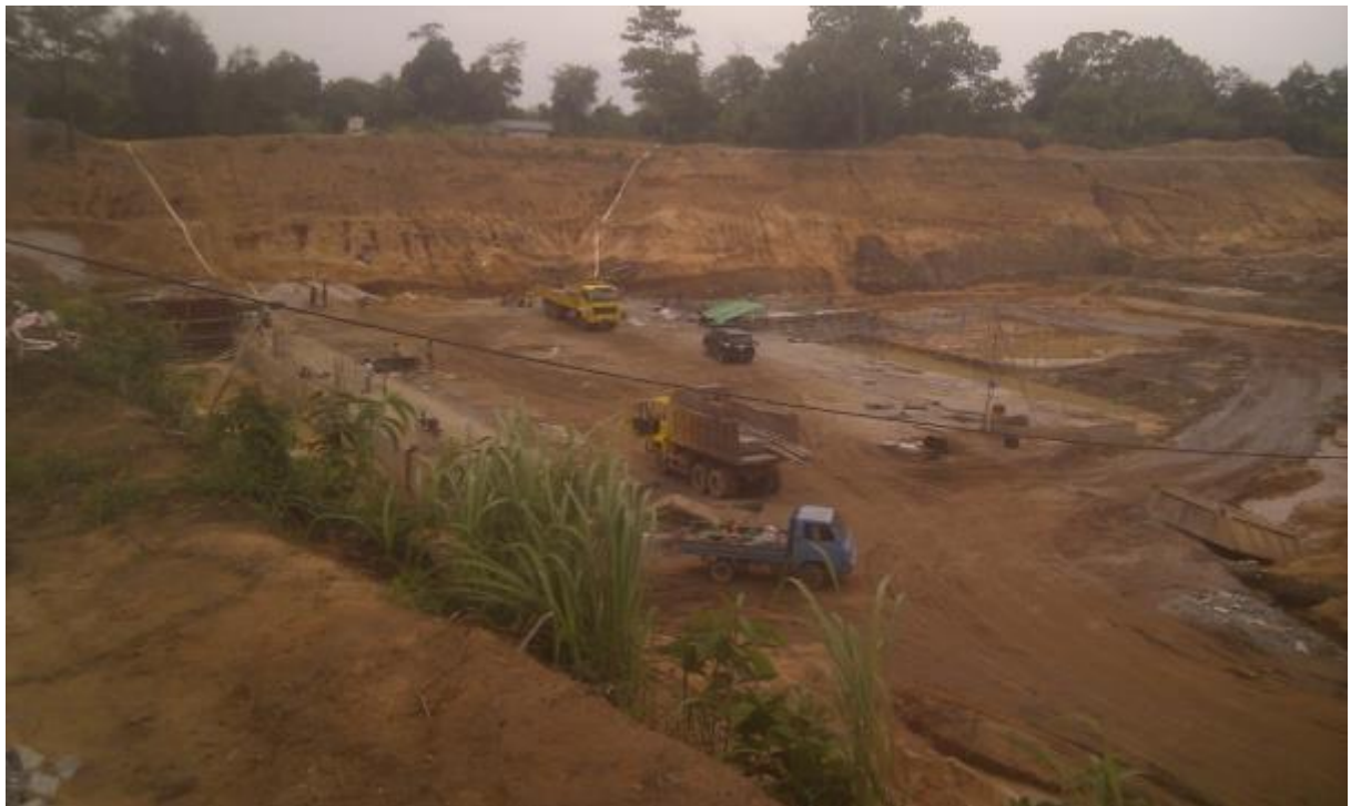
Figure 6.24 Construction of the Chinese Dam Near Srah Geov Village (November, 2015)
