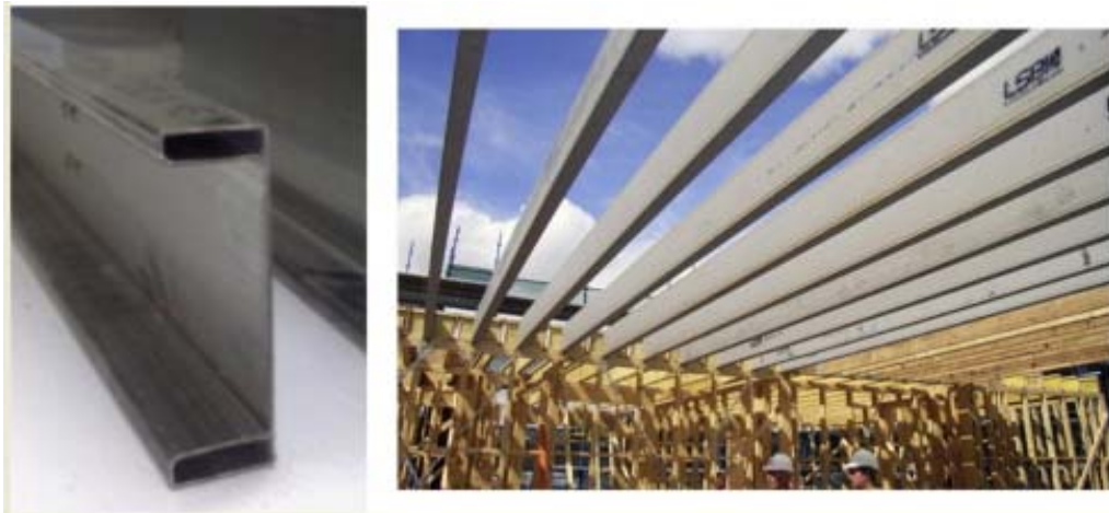
Figure 8.2: Channel section with hollow flanges
