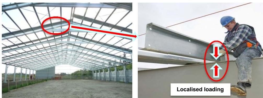
Figure 1.4: Localised loading
