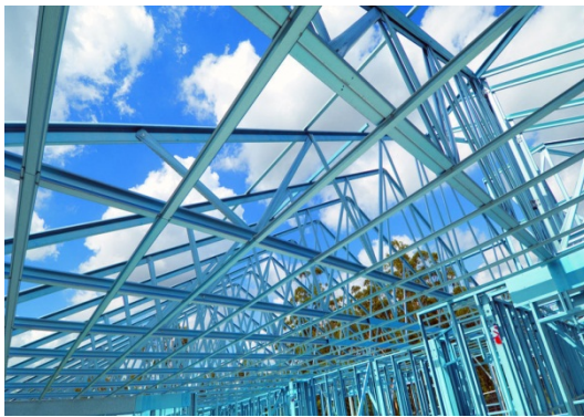
(a) Roof trusses
