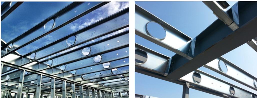
Figure 8.3: Cold-formed steel members with holes
