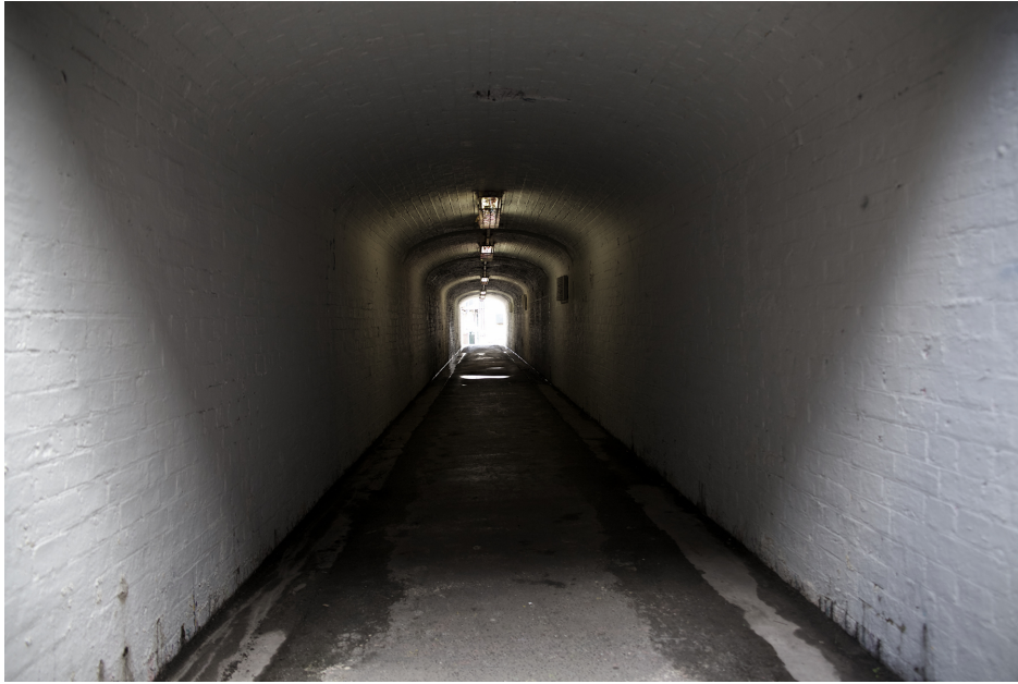
3.0 Newtown underground tunnel leading under the main railway line
