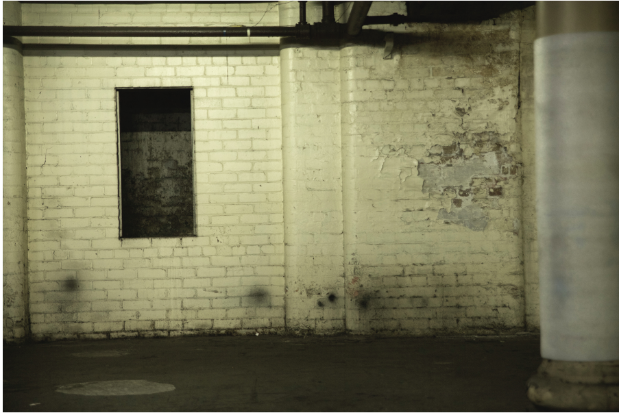
1.2 An example of Wynyard underground car park, Pitt Street, Sydney
