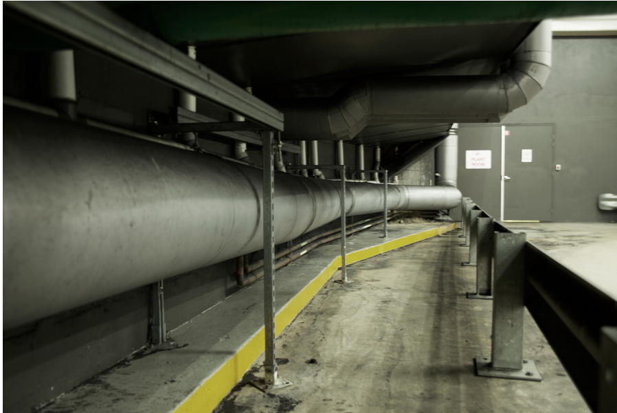
2.0 Entrance cavity to Queen Victorian Building underground car park
