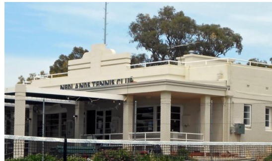
Functionalist/Art Deco: Nedlands Tennis Club, 1938, architects Harold Kranz and Neil Perkins, Bruce Street, Nedlands (N26) Photo: Graham Grundy, 27 October 2015
