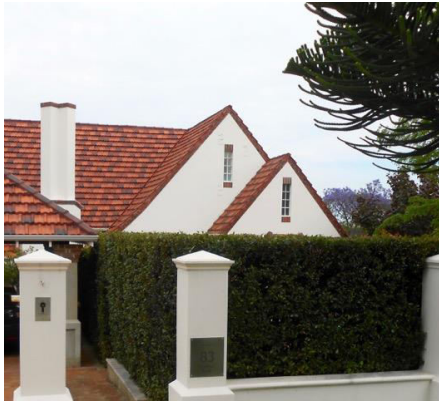
Old English: House, 1937, architect unknown, 83 Florence Road, Nedlands (N34) Photo: Graham Grundy, 27 October 2015
