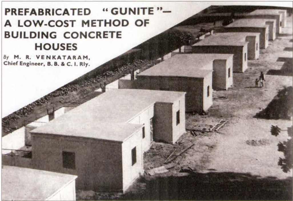
Figure 3.19 Prefabricated Gunitite workers housing at Delhi, 1950. 78
