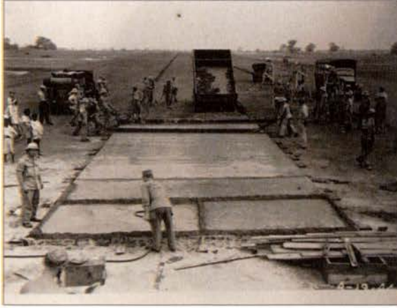
Figure 6.1 Albert Mayer's troops constructing an aircraft runway in Bengal near Kolkata. 13
