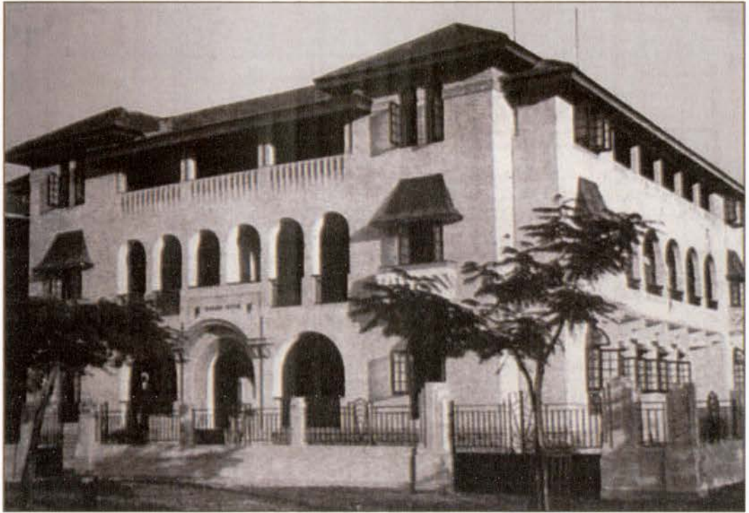
Figure 2.12 Baroda House, Multi storied apartment in Dadar-Matunga state. 40
