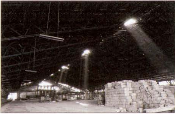
Figure 1.1 Inside the HHF's old factory. (Photograph Karim 2008)
