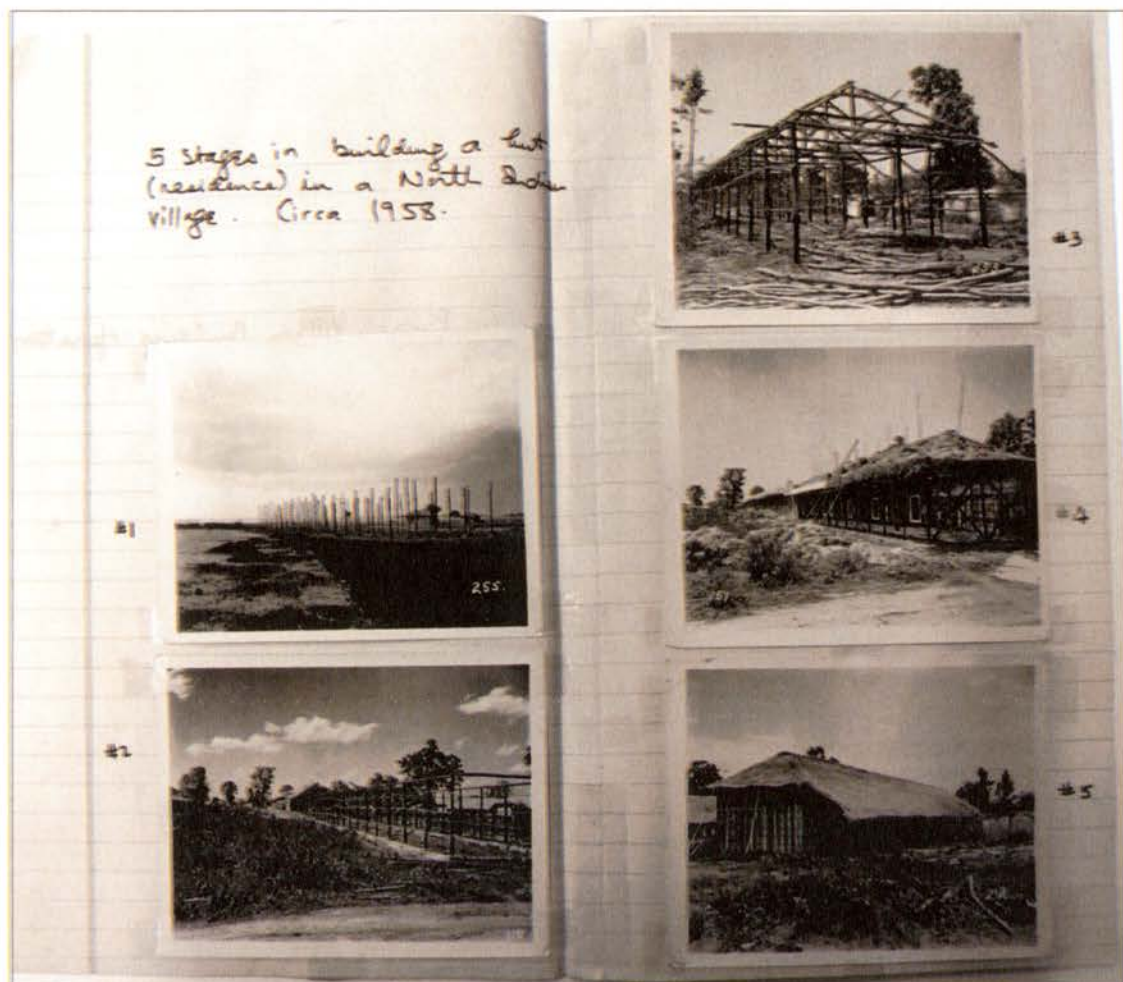
Figure 6.11 Images from Mayer's notebook: A study on the stages of rural hut construction, 1958. 46
