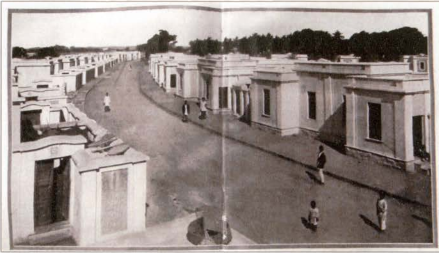
Figure 3.6 The workers quarter, built by HCB, circa 1914. 29
