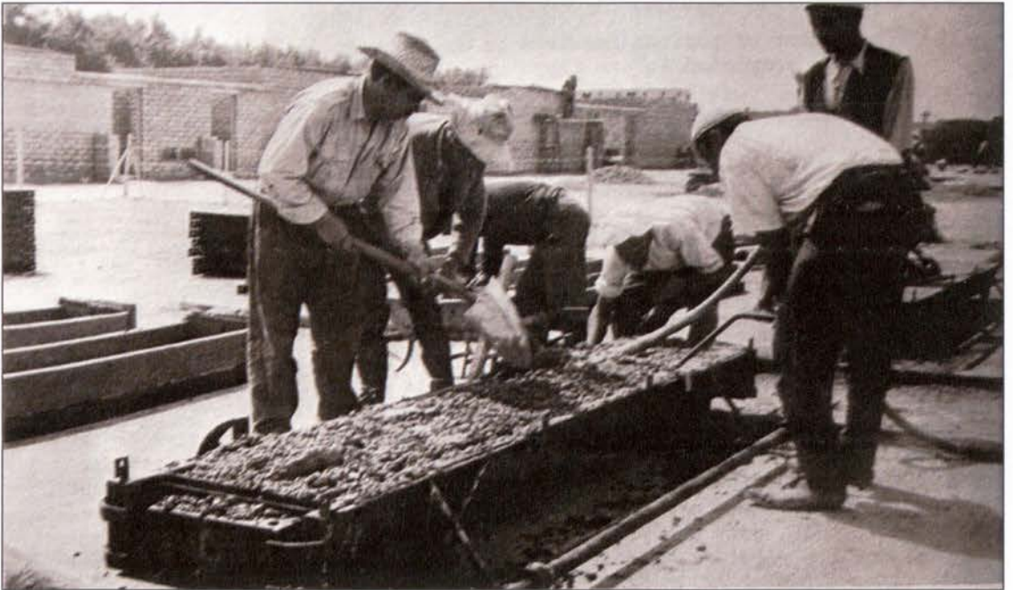
Figure 4.22 Construction of self-help housing. 80
