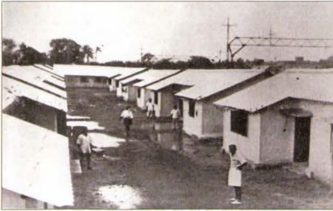
Figure 3.18 Railway Workers colony at Sen Nagar Santa Cruz, Bombay (1949). 75
