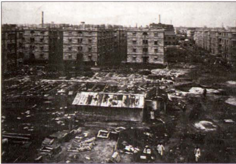
Figure 2.8 Worli Chawls under construction (n.d.). 28
