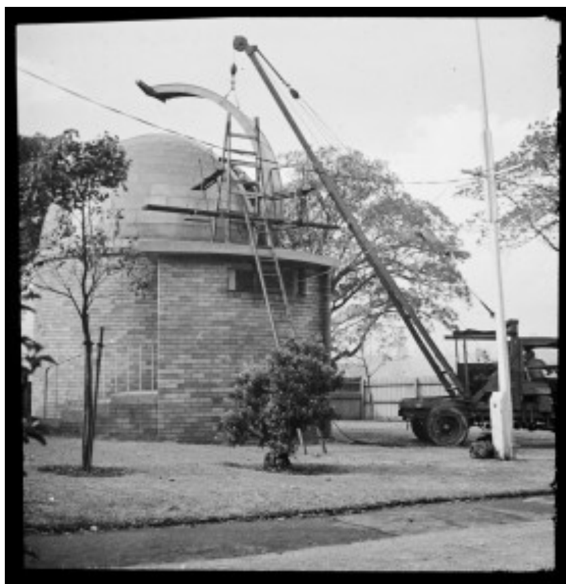
Figure 28: Astrograph House construction c1951 (Collection MAAS).
