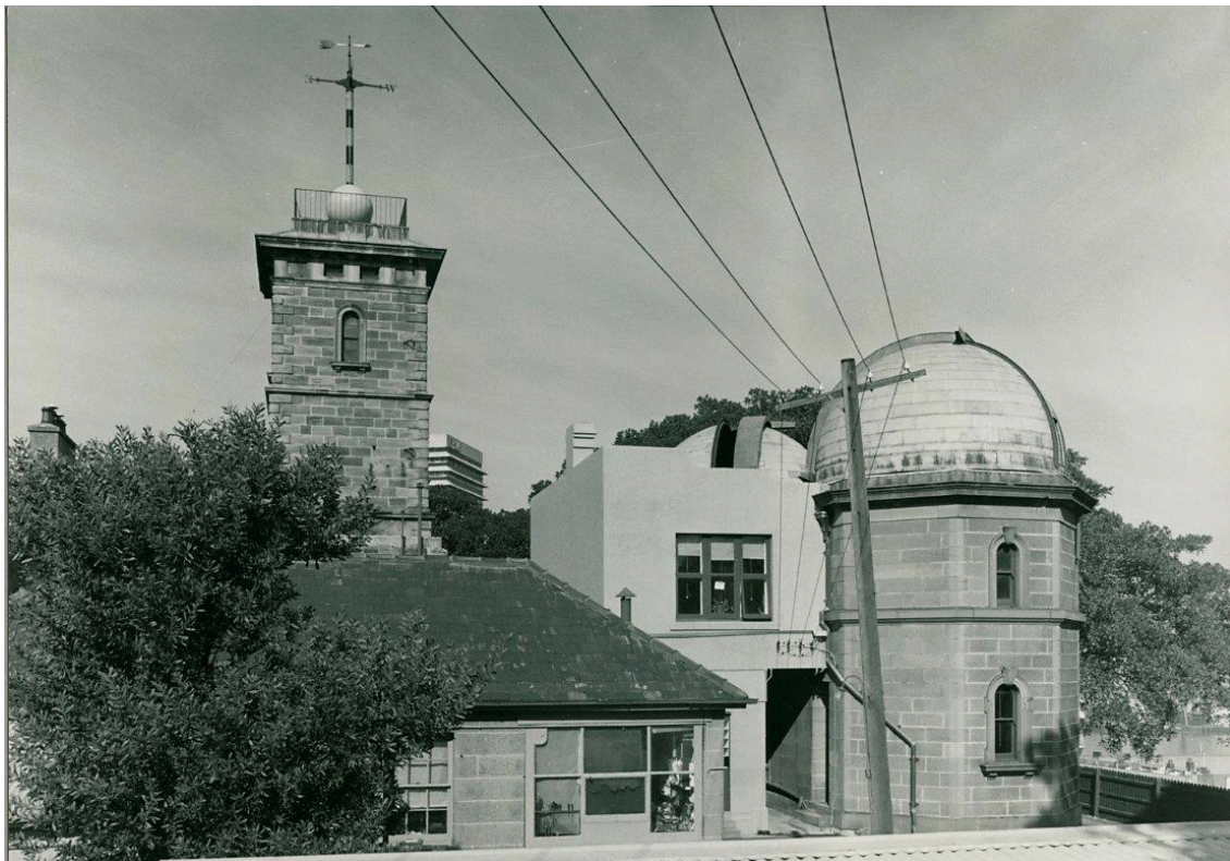
Figure 36: Sydney Observatory c1968, with the 1906 extension. Offices on the top floor were for the Measuring Bureau, switchboard and clerical duties (Collection MAAS P3549-216).
