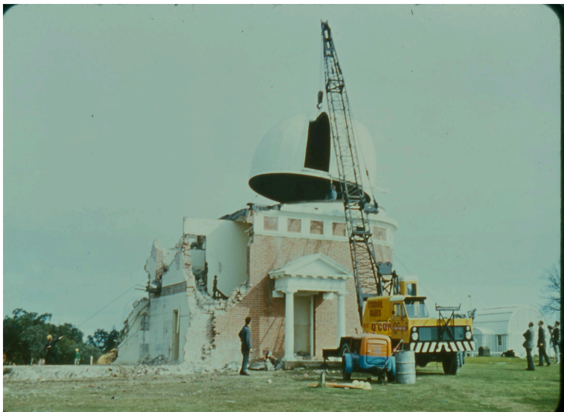
Figure 33: Demolition of the old astrograph house, 1964 (Collection Perth Observatory).
