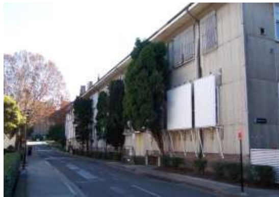
TRANSIENT BUILDING (F12) GFA 2,216 m 2 2 level, 1946 fibro building administration, laboratories, faculty
