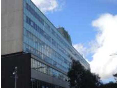
CARSLAW BUILDING (F07) GFA 17,022 m 2 , 8 level masonry & glass building
