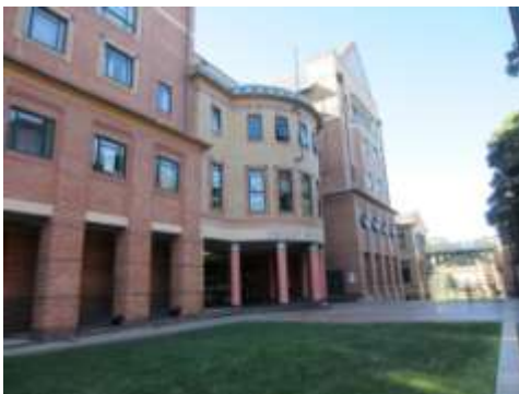
EDUCATION BUILDING (A35) GFA 10,138 m 2 , 9 level single brick building over concrete frame built 1993, lecture theatres, computer rooms, dance & drama studios, offices connected by elevated walkways to buildings A26 & A23
