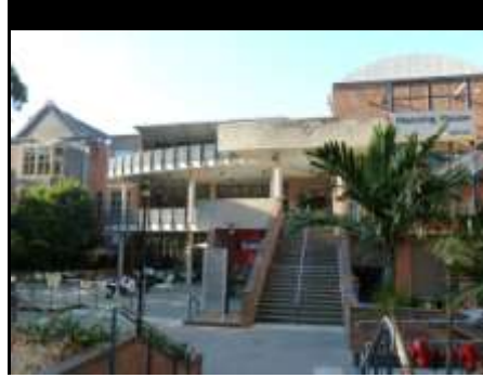
MANNING HOUSE (A23) GFA 3,952m 2 , 1914 heritage listed 2 level brick building, with 4 level extension (1999) bar, cafe, offices
