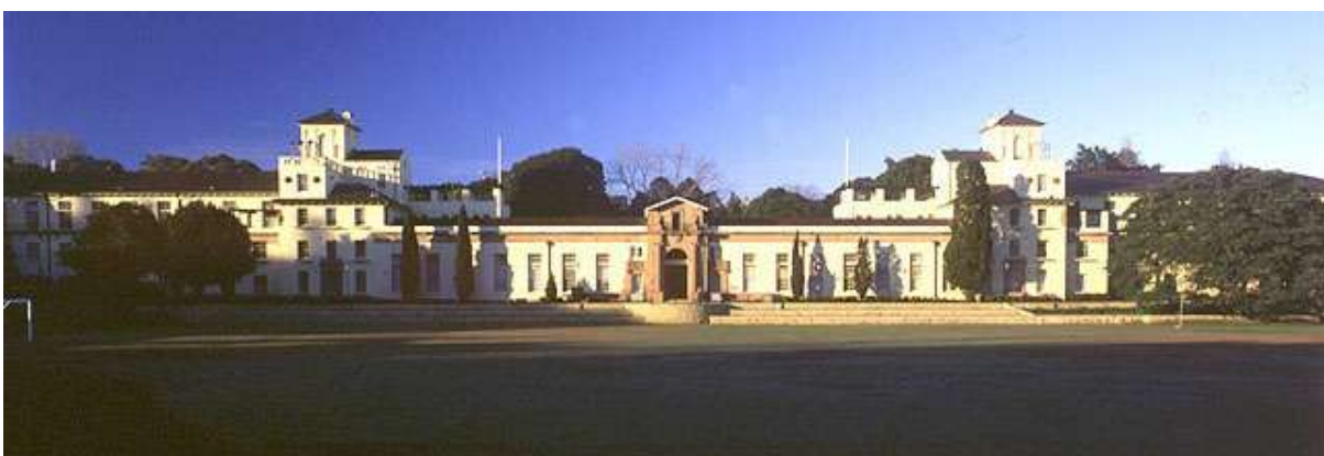
PHYSICS BUILDING (A28) GFA 8,404 m 2 5 level, 1940s masonry building – administration, teaching rooms, laboratories
