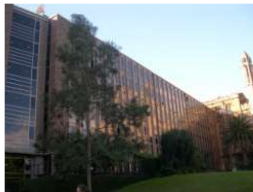
BRENNAN MACALLUM (A18) GFA 7,500m 2 9 level (refurbished 1990) masonry building administration, faculty staff in cellular offices, general access computer laboratories
