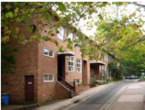
VICTOR COPPLESON/QEII (D02) GFA 1,219 m 2 2 level, 1940s masonry building administration, small laboratories
