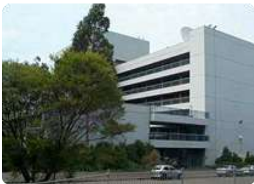
ELECTRICAL ENGINEERING (J03) GFA 9,396 m 2 11 level masonry, 1960s building, laboratories, administration, workshops
