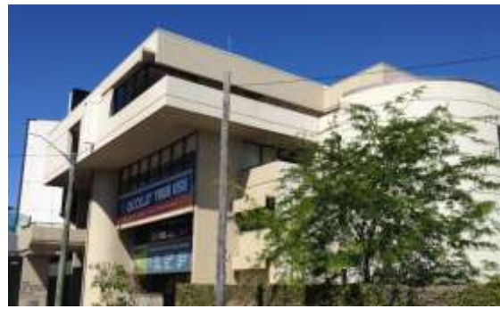
WENTWORTH BUILDING (G01) GFA 10,399 m 2 , 1960s masonry & glass structure, 6 level building with extensions in the 1970s and 1990s.
