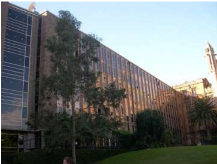
Figure 3 Brennan MacCallum Building at the University of Sydney, gross floor area 7,500 m 2 , with energy use of 53.0 kilowatt hours per square metre per annum (Table 4)
