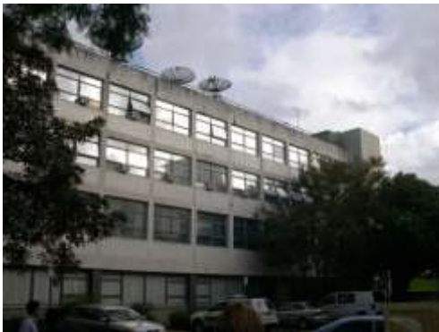
PHYSICS ANNEXE (A29) GFA 1,1738 m 2 4 level, 1960s light construction, administration and laboratories (since demolished and rebuilt)
