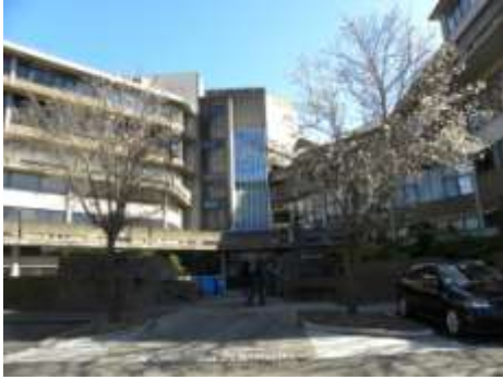
WILKINSON BUILDING (G04) GFA 11,313 m 2 6 level building, era 1960s, administration, lecture rooms, studios, workshop, cafe
