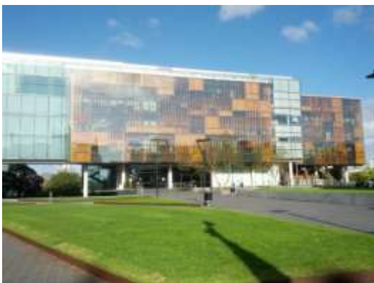
LAW BUILDING (F10) GFA 30,069 m 2 2009 built, concrete frame, steel and high performance glass facade, 2 basement car park levels with 6 floors above, lecture and seminar rooms, computer labs, library, cafe, offices
