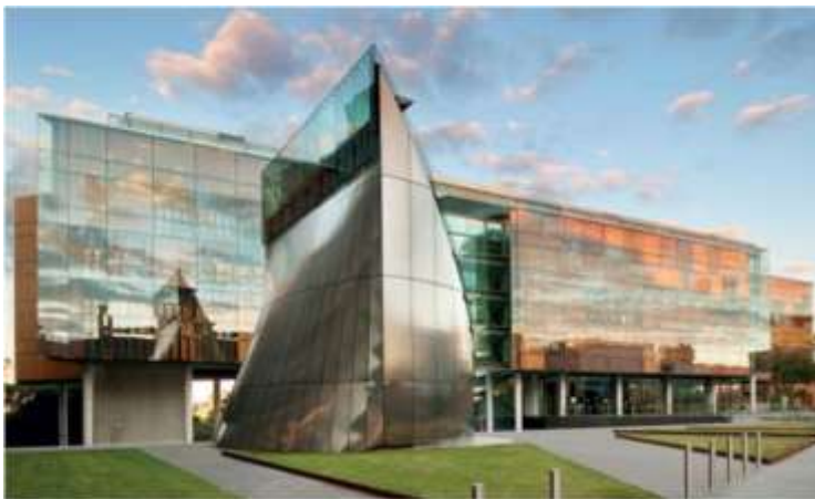
Figure 1 Law Building at University of Sydney, gross floor area 30,069 m 2 , with energy use of 91.1 kilowatt hours per square metre per annum (Table 4)
