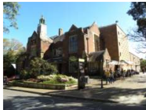
HOLME BUILDING (A09) GFA 6,760 m 2 5 level heritage listed, masonry student facility and recreation, with contemporary extensions - dates from 1913
