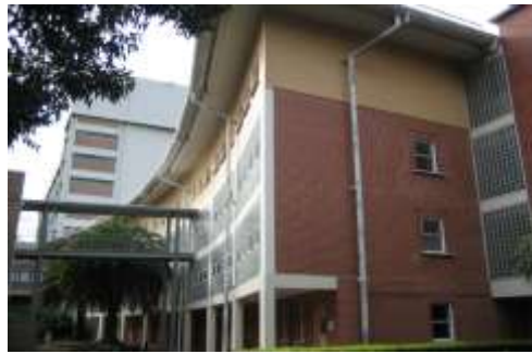
LINK BUILDING (J13) GFA 3,844 m 2 5 level, 1980s masonry building administration, lecture rooms, laboratories
