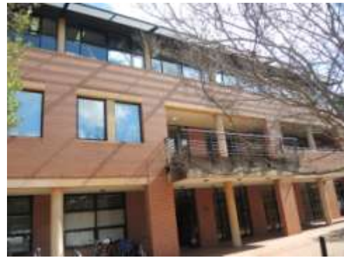
VET CONFERENCE CENTRE (B22) GFA 1,939 m 2 3 level masonry building, conference rooms, foyer, offices, service rooms, classrooms, meeting rooms, lecture theatre
