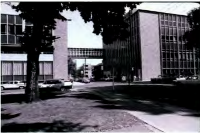
Aug 15, 1966: The Skybridge connects Portland State College Center (SMSU) and South Park Hall (Neuberger). Neuberger seems to be missing half of its building on the Broadway side.
