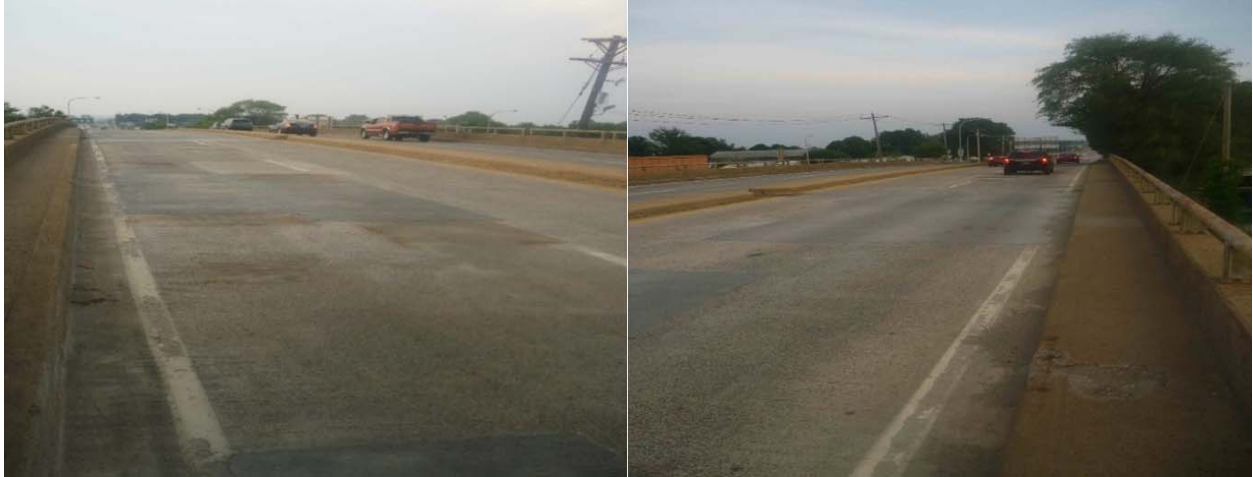
Figure 12. Bridge deck from both sides of approaching traffic.
