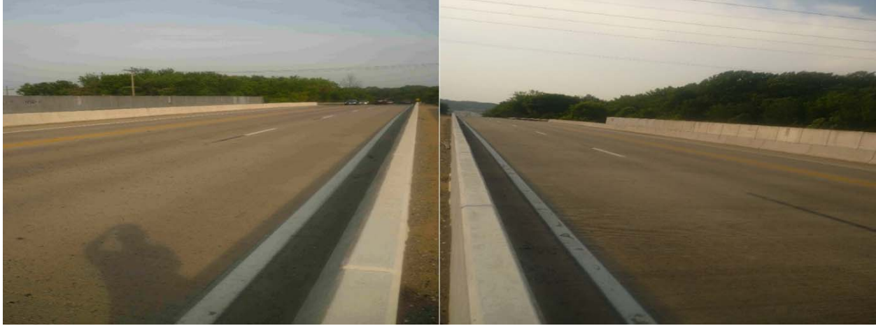
Figure 8. Bridge deck from both sides of approaching traffic.
