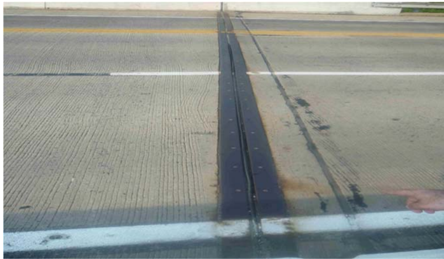
Figure 9. Approach slab and joint.
