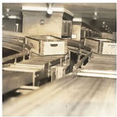
Step 7. The box with the requested book winds its way through the Bookstacks toward the Main Reading Room of the Central Library of the Free Library of Philadelphia
