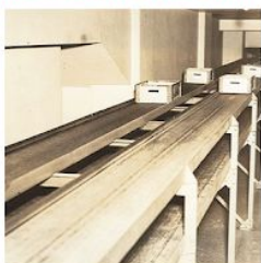
Step 8. Eventually the box with the requested book makes its way to the sixth level of the Bookstacks and across the first mezzanine floor to a point directly under the Main Reading Room of the Central Library of the Free Library of Philadelphia
