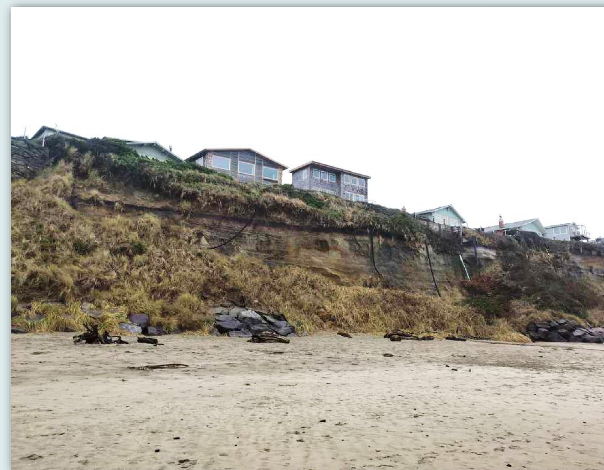
Figure 3: Photo from Road's End, Lincoln City showing signs of erosion. The sandstone sea cliff is visibly oversteepened, houses sit dangerously close to the edge of the cliff, and riprap can be seen in a couple of places.
