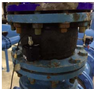
Figure 3. Stretched single ball rubber isolator.
