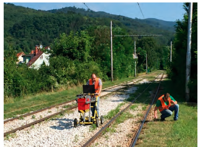
Fig. 7. Conduction of GPR investigations for the tram embankment condition assessment [10]
