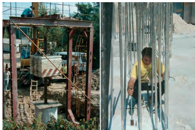
Fig. 1. Dynamic testing of the pile capacity and integrity of pile columns
