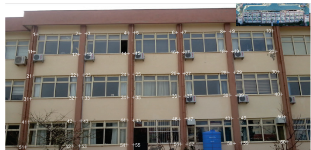
Figure 8 60 corner points on the building facade and 3D model of the same facade at the upper right corner.
