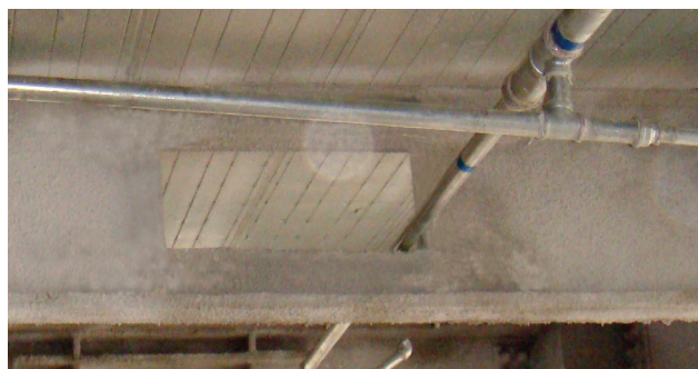
Figure 1 Composite beam with web opening
