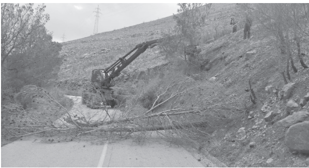
Fig. 2 Removal of fired Aleppo pine biomass from fire site
