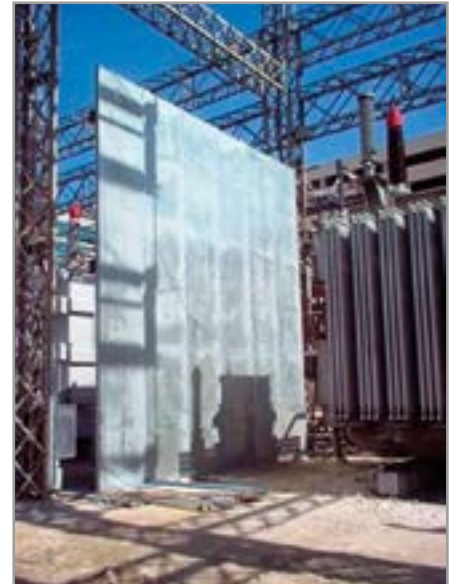
Figure 9. Local CIP using proximity ballistic fire barriers
