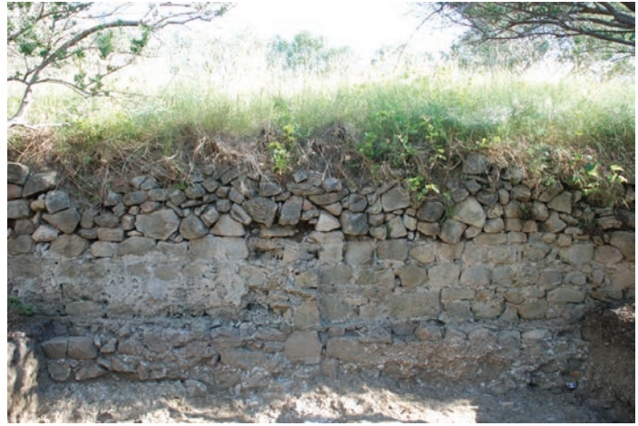
Fig. 5. Northern wall of the church during excavation (photo: F. Giacomello).
