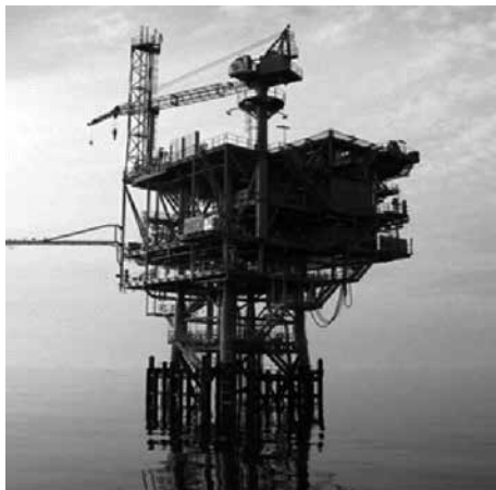
Figure 8 Gas platform Marica
