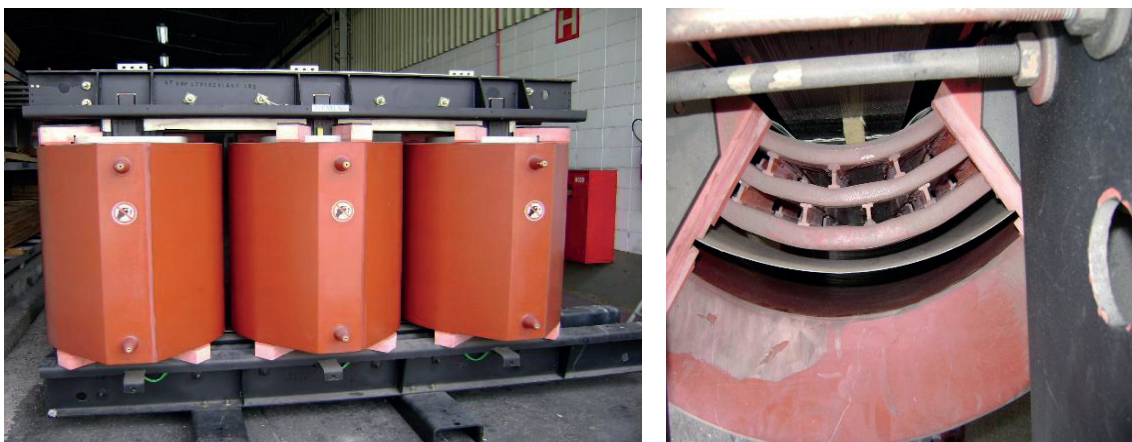
Figure 5 – Side and top views of cast resin transformer without enclosure
