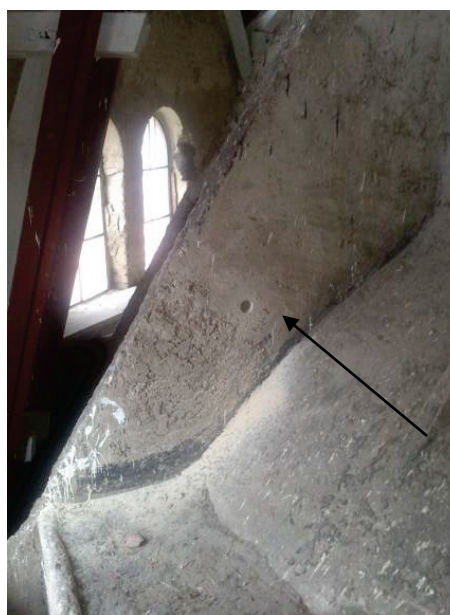
Figure 9 Sampling of concrete from the dome in Subotica Synagogue
