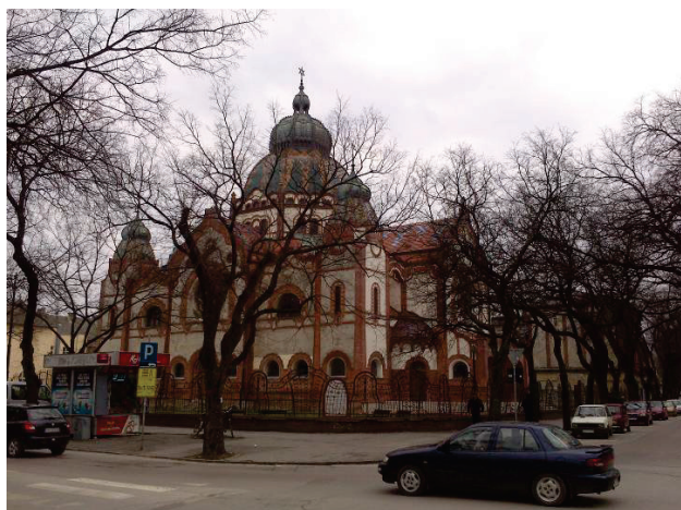
Figure 3 The walls of the Subotica synagogue are made of brick masonry and the foundations of stone
