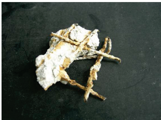
Figure 8 Corrosion of steel in concrete sample from synagogue in Subotica
