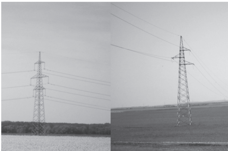
Figure 2. The two pylon types in the Baranya area: left type A („bačva“) and right type B („jela“). (Photo: A.Tomik)
