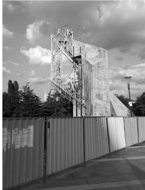
Figure 6: The Demolition, July 14 2017. Photo: Valery Gyurov. Source: Facebook
