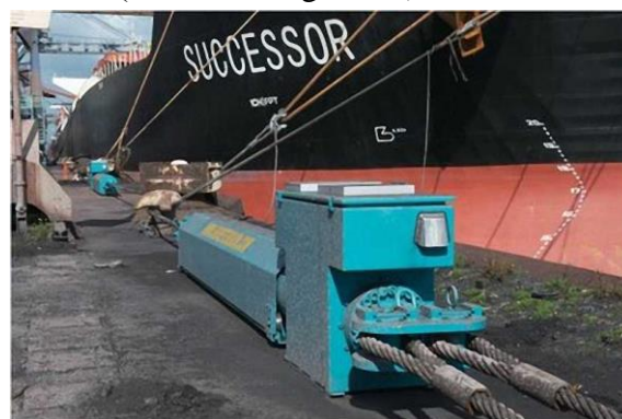
Fig. 12 – Hydraulic mooring system. Source: KRVE (2016)
