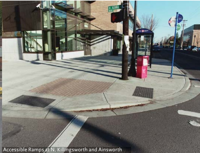
Accessible Ramps at N. Killingsworth and Ainsworth
