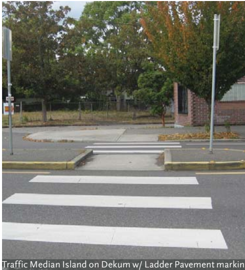
Traffic Median Island on Dekum w/ Ladder Pavement marking
