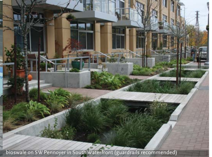
bioswale on SW Penoyer in South Waterfront (guardrails recommended)
