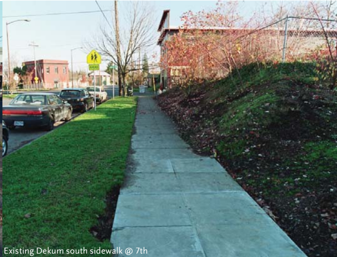
Existing Dekum south sidewalk @ 7th
