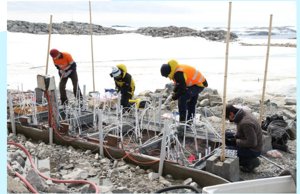
Casey Station Contaminated Site: Use of Permeable Reactive barrier to remediate soils (antarctica.gov.au, 2014)
