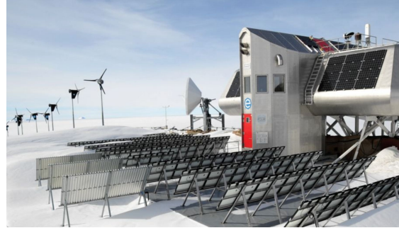
Belgium's Princess Elisabeth station and its solar and wind infrastructure. http://www.antarcticstation.org
