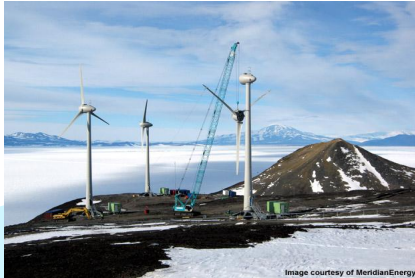
Ross island wind farm construction in 2009. Image credit Meridianenergy.co.nz
