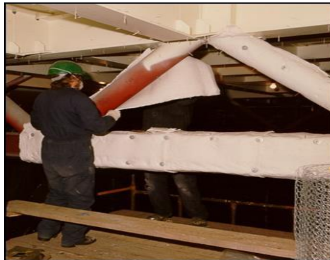
Figure 2.6. Application of blanket fire protection on structural steel members (SCI, 2016).
