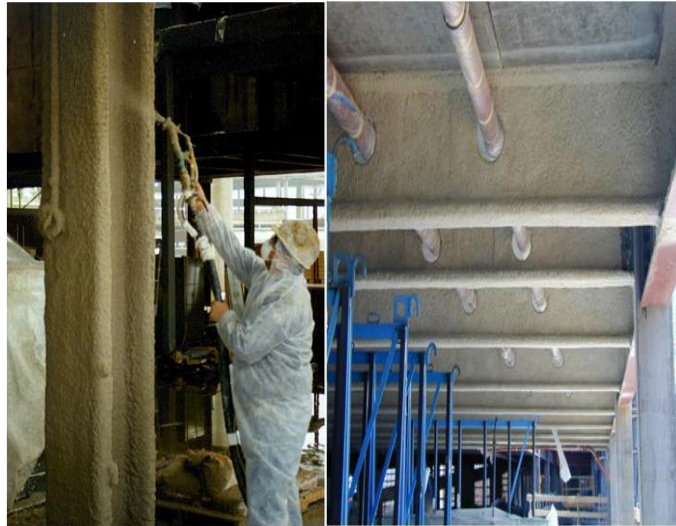
Figure 2.4. Cementitious spray application (SCI, 2016).
