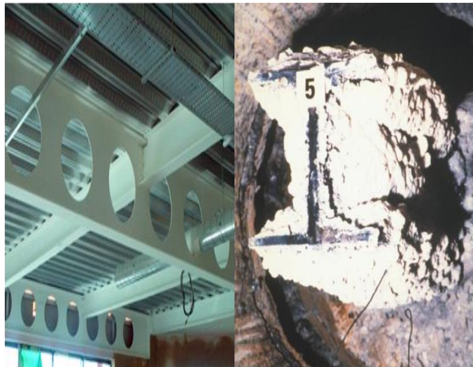
Figure 2.5. Finished application of intumescent coatings and the result of intumescence (SCI, 2016).
