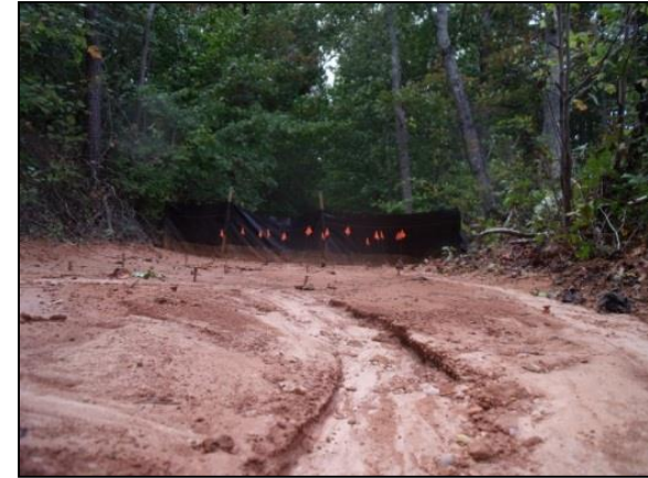
Silt fence barriers and erosion pin networks were installed to trap and measure sediment delivery.
