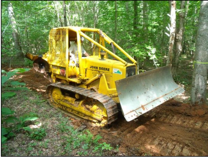
Bulldozer blading to reopen legacy road approaches.
