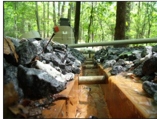
Open-top box culvert
