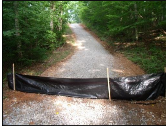
Silt fence barriers and erosion pin networks were installed to trap and measure sediment delivery.
