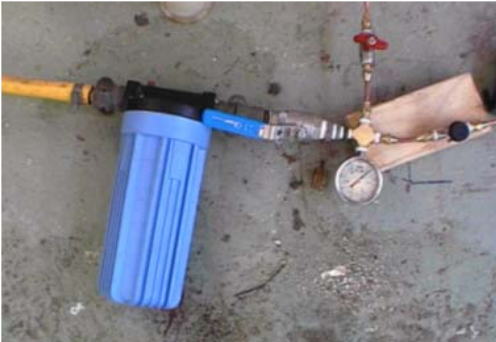
Figure 34 - Water filter, pressure gage and control valve
