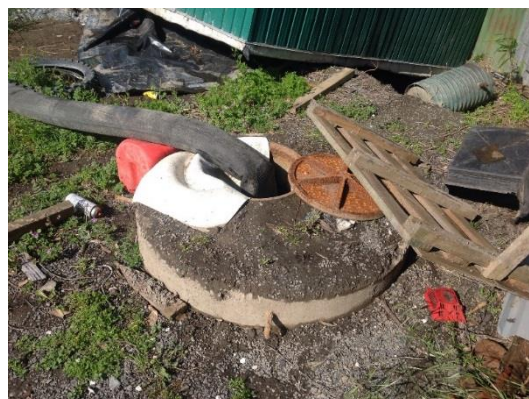
Figure 33: Floatation of manhole on Beach Road near to Lyell Creek ( -42.3848^\circ , 173.6783^\circ taken facing SW).
