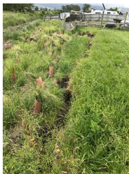
Figure 34: Lateral ground movements associated with vertical settlements in grassy area between Beach road and Lyell Creek. Note: Cracks are associated with vertical offsets and blocks have rotated away from the creek ( -42.3902^\circ , 173.6777^\circ , taken facing N).
