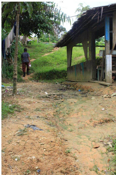
Figure 6. 4 The evacuation route is steep to climb and eroded from the rain in Dusun Passibut Source: Personal documentation taken during the field study
