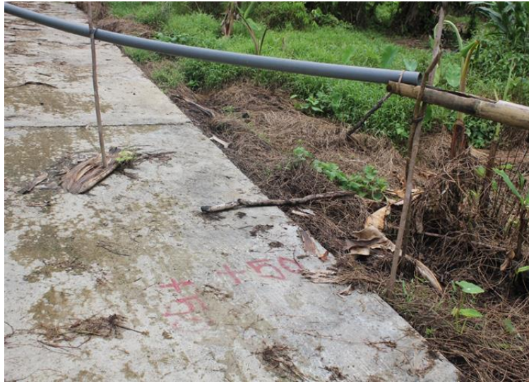
Figure 6. 3 The evacuation route was blocked by a water pipe to flow clean water the several households nearby in Dusun Makukkuet Source: Personal documentation taken during the field study
