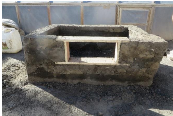
Figure 4.3.8.3: Detail of wooden frame for solar cooker drawer
