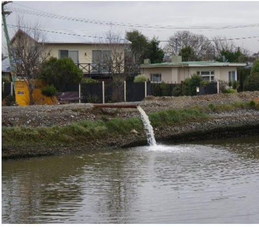
a) Raw sewage discharging to Avon/Otākaro River upstream from Owles Terrace sampling site
