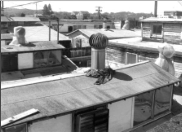
Chiquita rooftops. Photo by A. Van Asperdt
